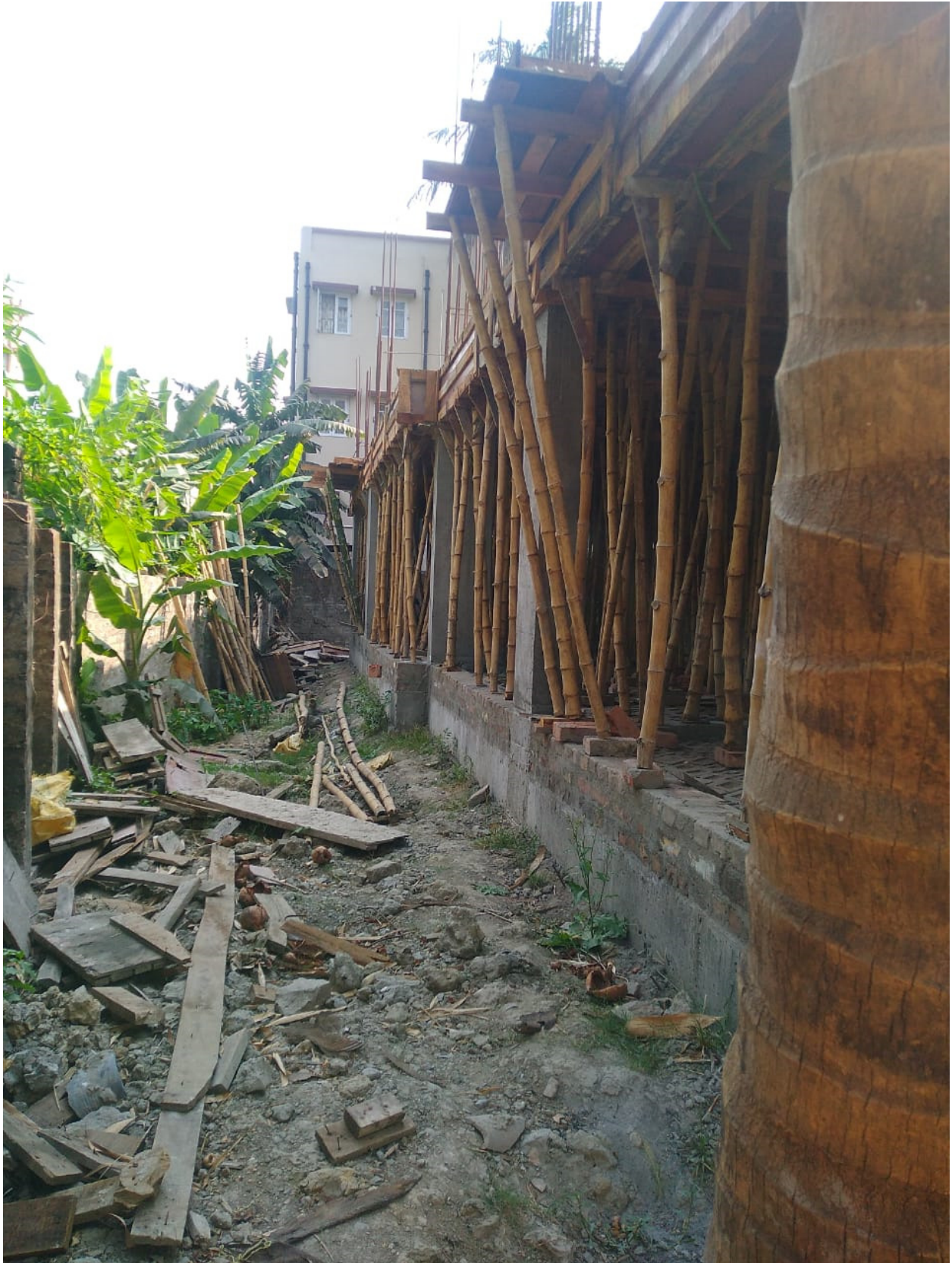
GLOBAL RESIDENCY_GROUND FLOOR ROOF CASTING UNDER PROGRESS
